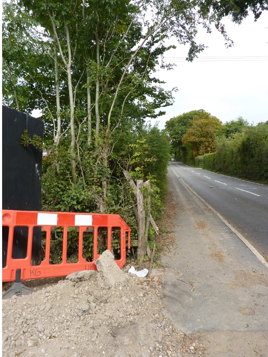
Line of existing hedge, wire mesh fence just visible in centre
